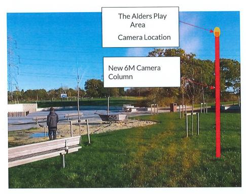
The proposal for mounting the  $2 \times CCTV$  surveillance camera within The Alders Play Area would be to install a new 6m column and associated power. Note due to the location of the play area, there is limited access to local mains power.
