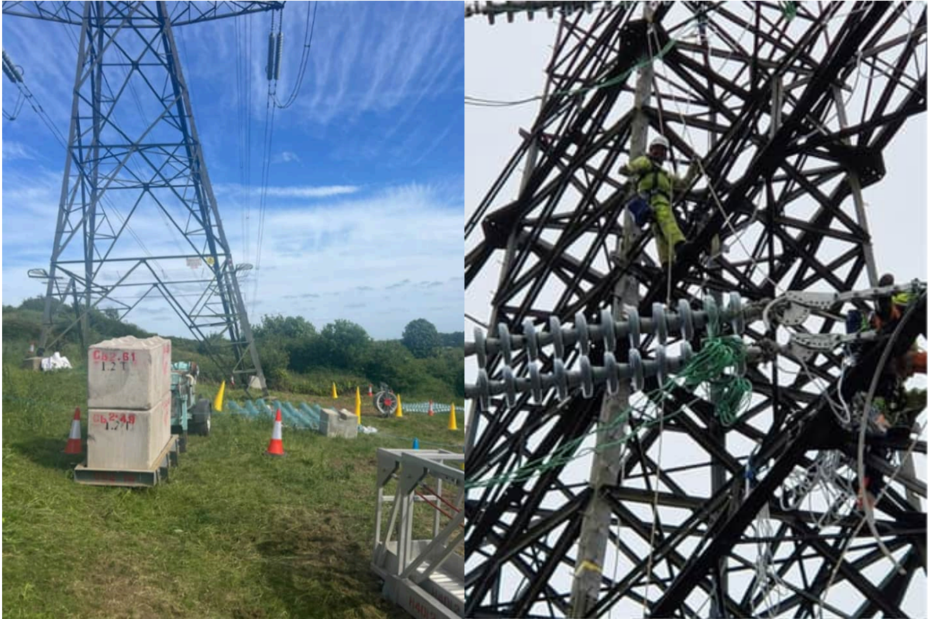
Site set up on the Lovedean to Bolney Overhead Line route in preparation for raising the working platform. The new insulators are positioned on the ground, prepared to replace the existing insulators on the pylons.
